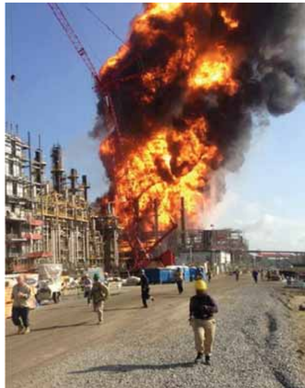
Bild A6-12: Gaswolkenexplosion (Quelle: U.S. Chemical Safety Board (CSB); http://www.csb.gov/ )
