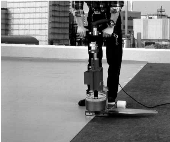
Fig. 6: Thermal insulation – mechanical fixing
