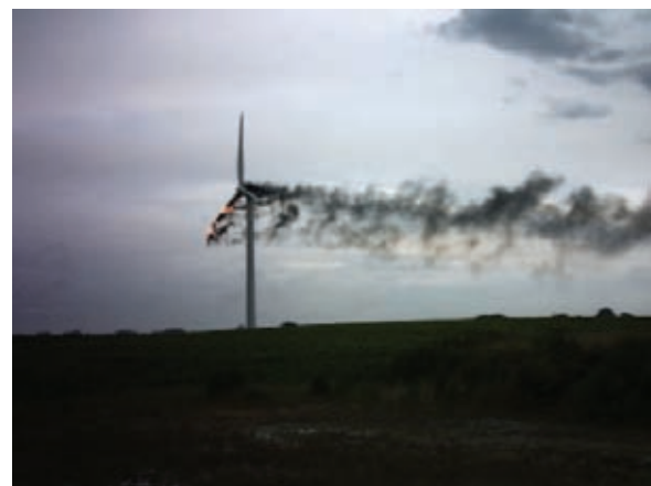
Fig. 1: Fire after lightning struck a 2 MW wind turbine in 2004 (Image source: HDI/Gerling)
